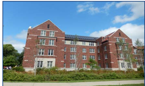
Rooftop Solar, CERTs
