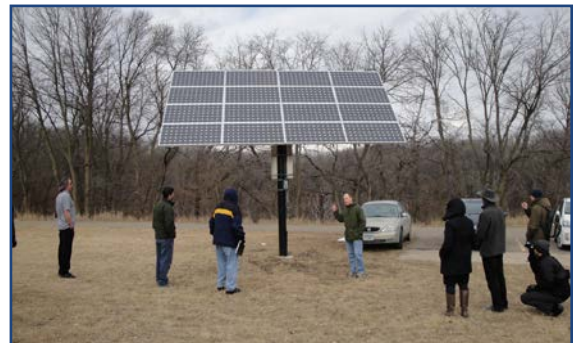
Ground Mount System, CERTs
