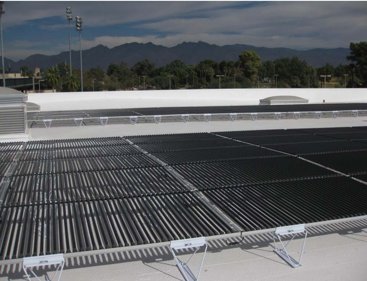
Cylindrical Solyndra PV panels are installed on top of the City Parks Warehouse in Tucson, Arizona. (City of Tucson /PIX18041)
