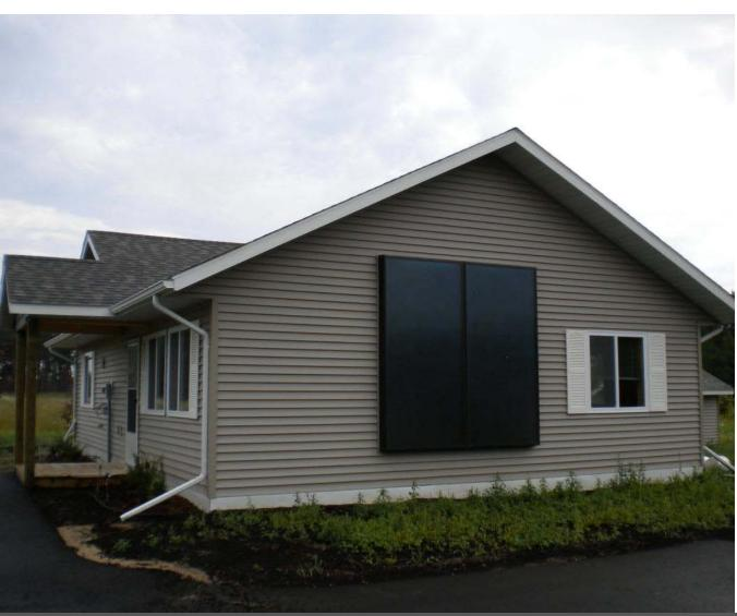
Provides heat by recirculating conditioned building air through solar collectors
