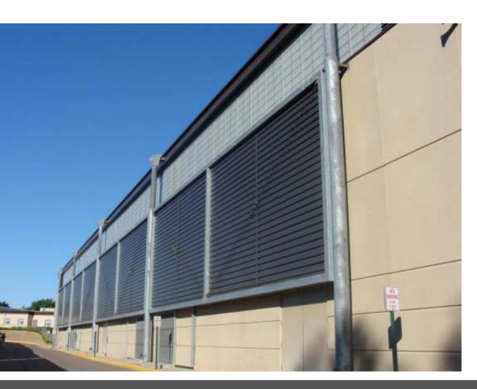
Preheats incoming building air using solar radiation captured by solar walls (unglazed transpired collectors)
