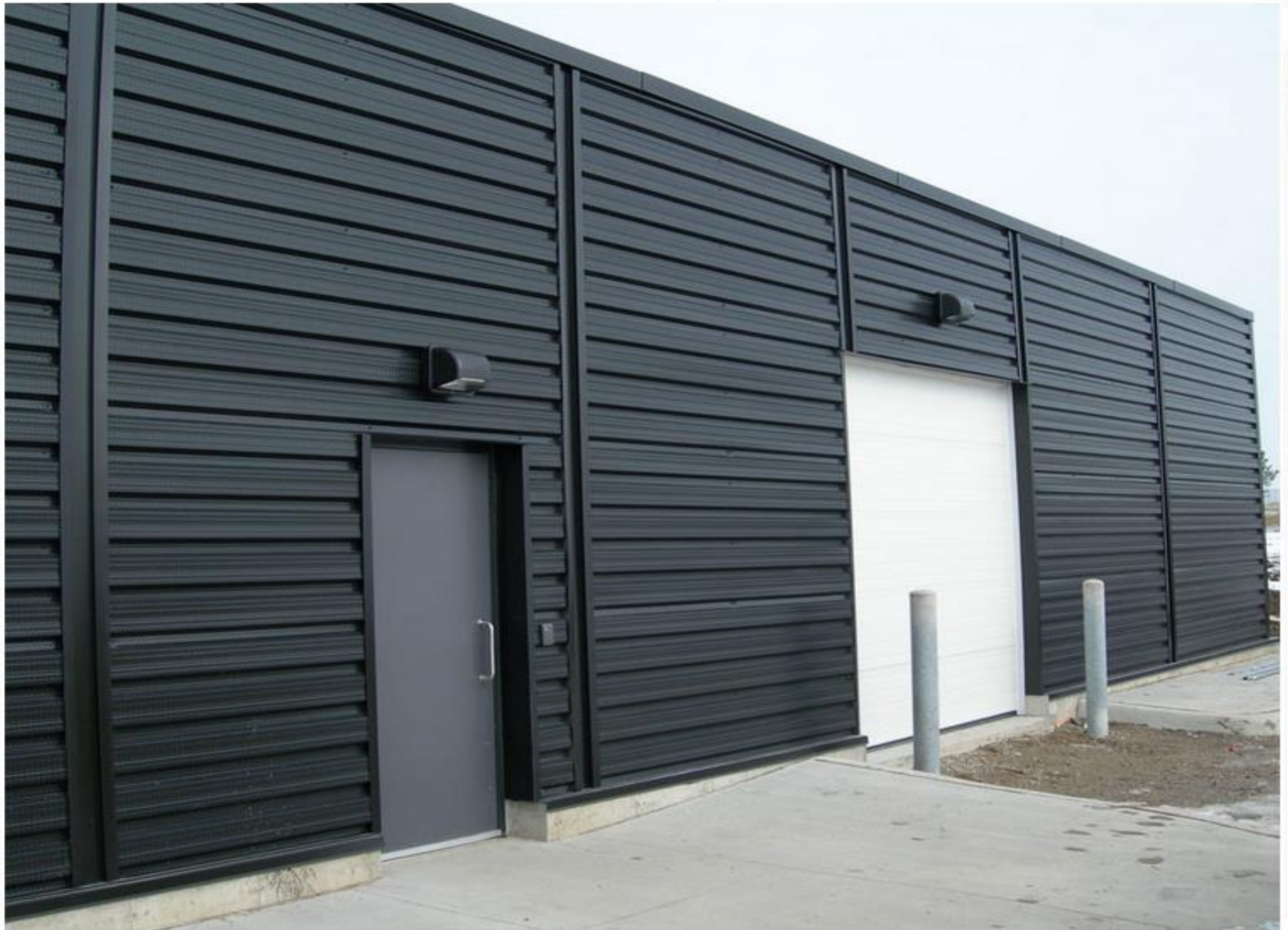
Waterloo Police Station, ON - Canada
