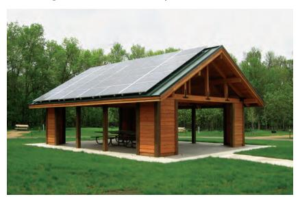
Minnesota's Department of Natural Resources has installed a 13.8 kW roof-mounted photovoltaic system on a picnic shelter in a new campground at Lake Shetek State Park.
