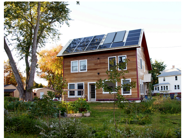
The Giordano---Smeltz Zero Net Energy residence.
