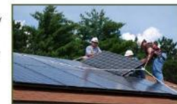
Rooftop Solar, MRZA
