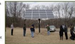
Ground Mount System, CERTS
