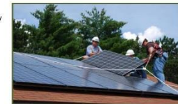
Rooftop Solar, MRCA
