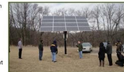
Ground Mount System, CERTs
