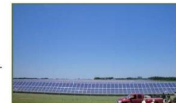
Solar Farm, CERTs
