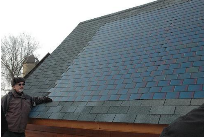
Figure 10: BIPV system, solar PV panels are built into the shingles of a roof ( http://solarenergyfactsblog.com )
