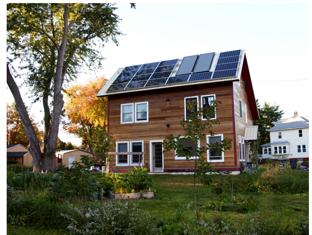
The Giordano-Smeltz Zero Net Energy residence.
