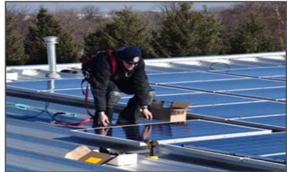
Rooftop Solar, Parkland Community College, IGEN
