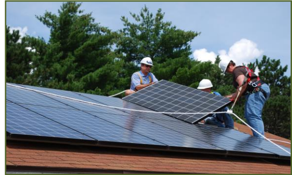
Rooftop Solar, MREA
