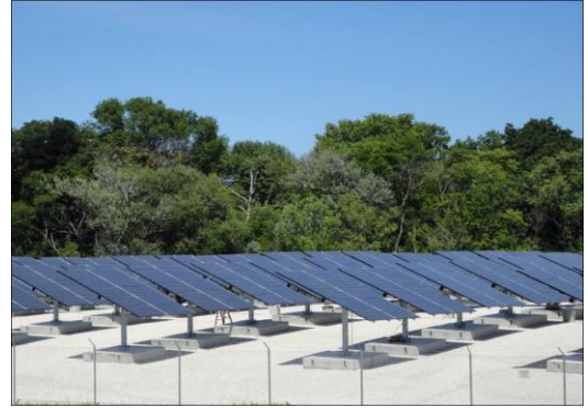
Solar Farm - MATC Blue Hole Project Located on Capitol Drive in Milwaukee.
