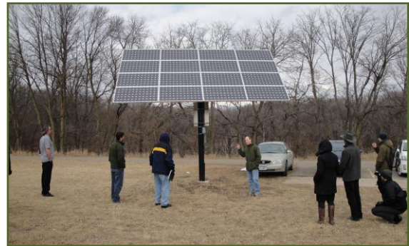
Ground Mount System, CERTs
