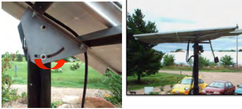
Adjustable and Tracking Arrays may require flexible wiring methods.
