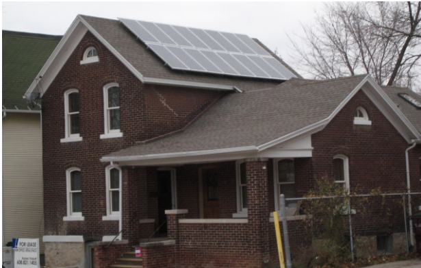
Photo 1. A 2.8 kilowatt (kW) solar electric system mounted flush to the roof of a historical building in Madison, Wisconsin. No other roof area was well suited to the solar electric system (photo credit: Niels Wolter, Focus on Energy).
