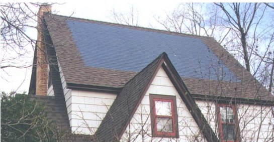
Photo 3. Solar electric shingles (made by UniSolar) with a capacity of 1.6 kW on an older home in Madison, Wisconsin (photo credit: Niels Wolter, Focus on Energy).
