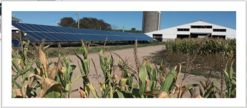
25KW SYSTEM IN FALMOUTH, MICHIGAN
