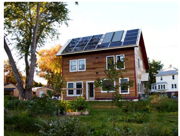
The Giordano-Smeltz Zero Net Energy residence.
