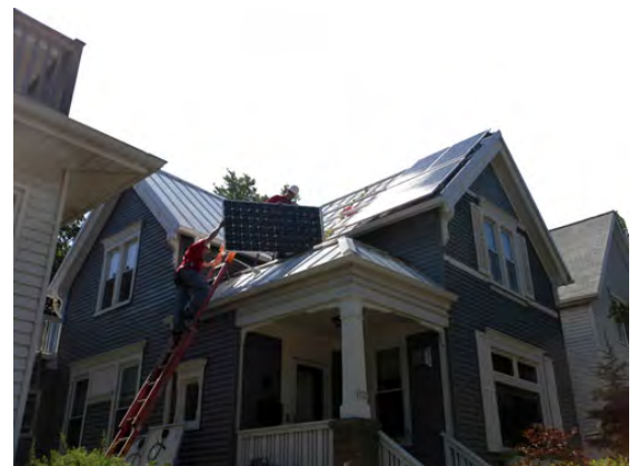
A Milwaukee solar group buy resident installation.
