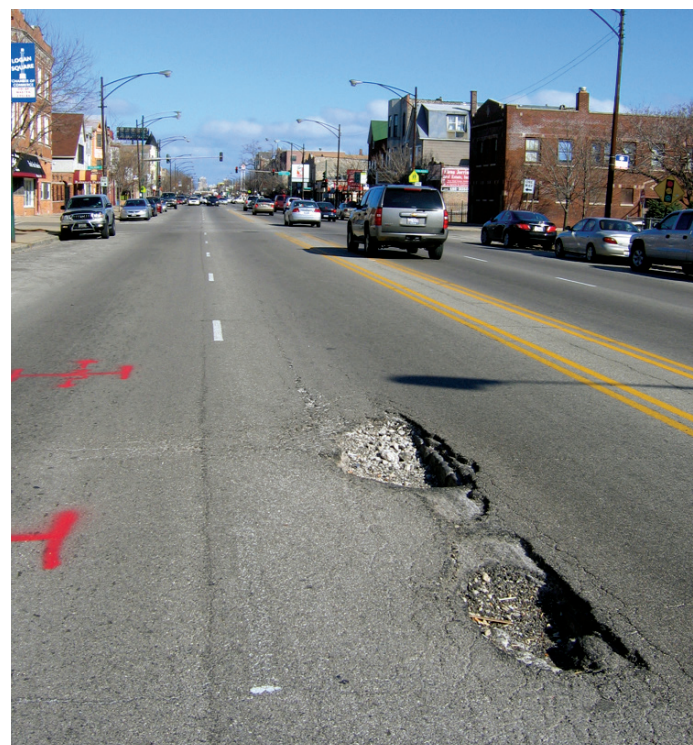
Rapid temperature fluctuations may accelerate pothole formation.
