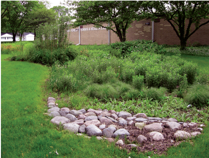
Green infrastructure, like this rain garden, can be used to capture runoff. Photo courtesy of Chicago Metropolitan Agency for Planning.
