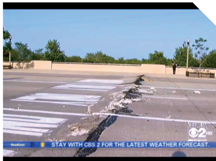
Pavement on Columbus Drive in downtown Chicago buckled during 103 °F heat in July 2012.
