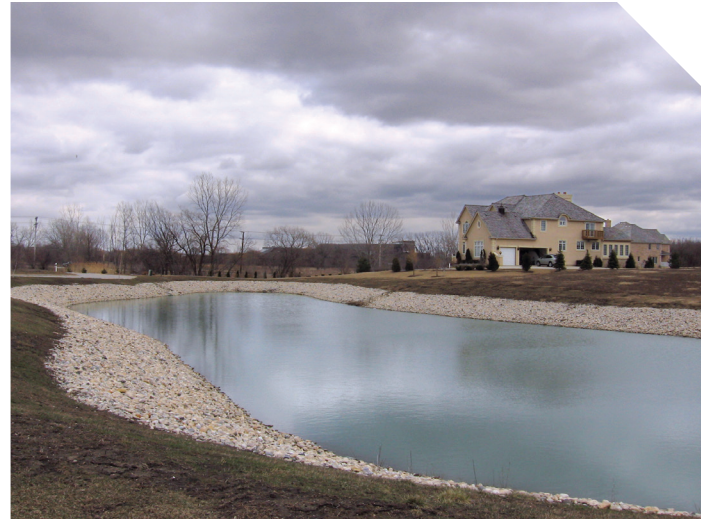
Detention basins, like this one in South Barrington, are designed to handle a certain design rainfall. These standards may need review to make sure they will provide adequate protection in the future. Photo courtesy of Chicago Metropolitan Agency for Planning.
