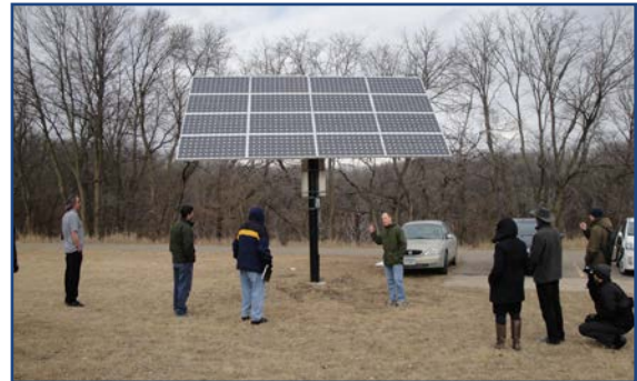
Ground Mount System, CERTs
