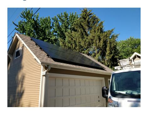
Pictured above is a 26 module, or 8.84 kW DC, solar array. Estimated annual solar production = **11,200** kWh
